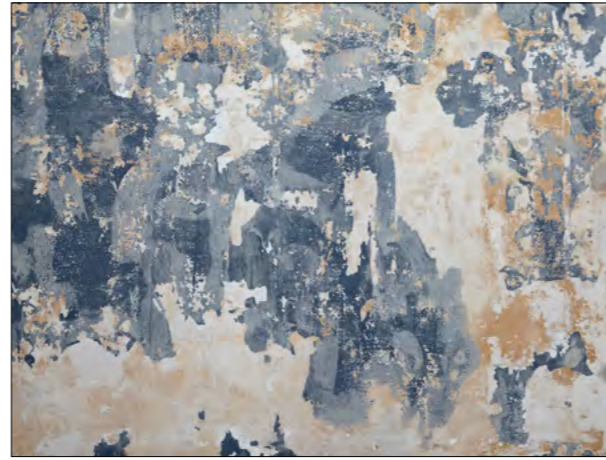
R12791 | BATTERED WALL R
