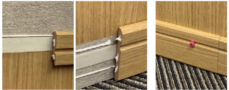
Apply adhesive to the sides.
